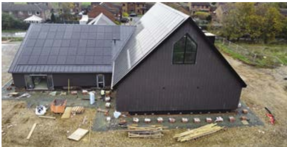
Things are progressing on the new community centre.
