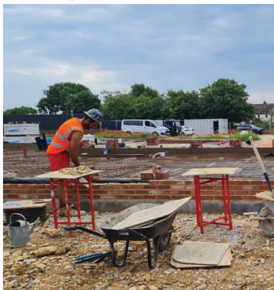
Building work progressing on the new community centre.
