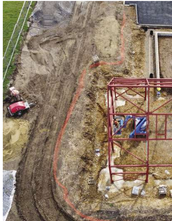
Aerial view of the Easton Community Centre construction.
