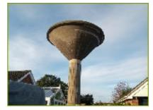
The Easton tower is a brutalist design in reinforced concrete so probably originates from 1950's. In the photo you can see three horizontal stripes where it looks like the concrete has had to be reinforced a bit more. They also help to give the impression of a thin lipped, narrow eyed sentinel scanning the Eastern sky.
